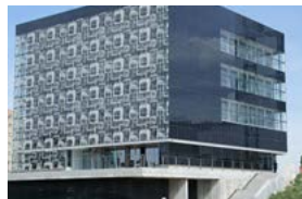
CIEM and CIRCE buildings Zaragoza (ES)
