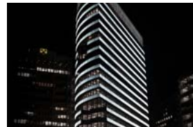
Raiffeisen Tower Vienna (AT)
