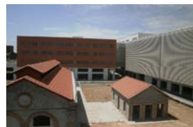
New office building of the Region of Central Macedonia, Thessaloniki (GR)
