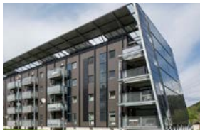
Retrofitting multi-family house Kapfenberg (AT)
